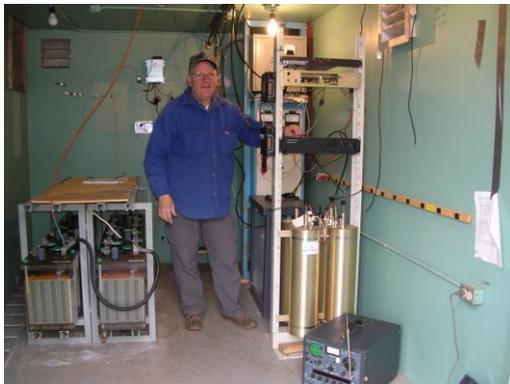
***Gary (VE7LCP) proudly showing newly installed 146.88 repeater, duplexer, charger (above his right shoulder) and link radios (mounted sideways on outside of rack).***
