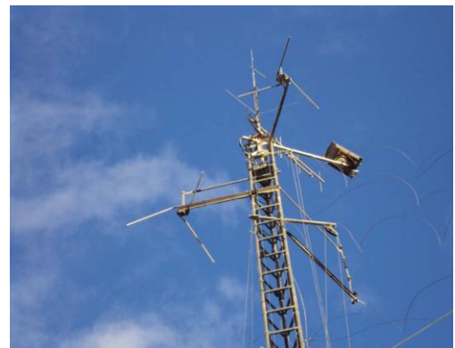
Ric's (VE7CUP) tower during installation of antennas and web cam.
